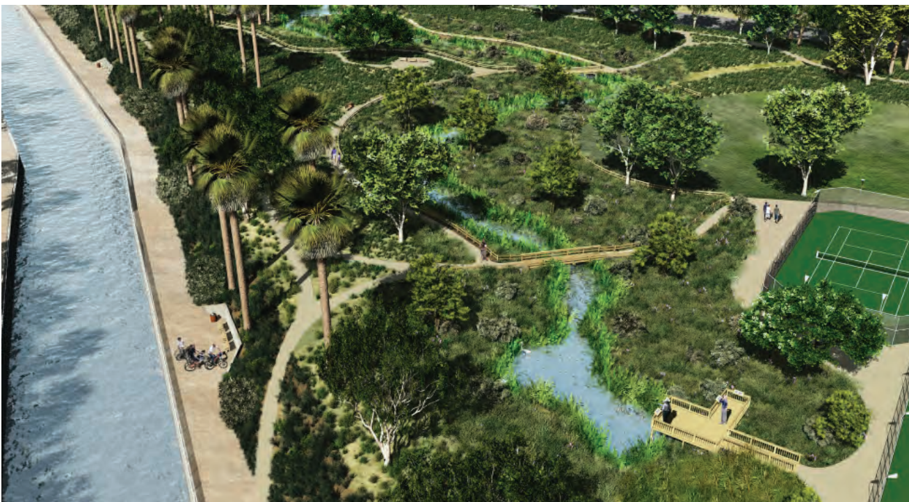
Naturally Improving Water Quality. Using a system of wetland habitats, the L.A. River Natural Park would use a "Green Solution" approach to naturally capture and clean polluted runoff from the surrounding urban area.
